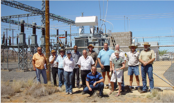
▶ A recent site inspection by the SKA SA team, along with some of its industrial and engineering partners.
